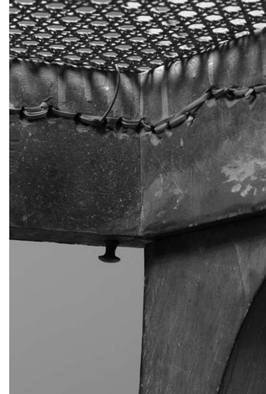
Figure 4 Inside of the proper left rear corner. Note the holes for the caning through the joints, the splashes of paint on the inside of the seat rail around the rear leg, the drips from painting the caned seat, and the scribe marks for the horizontal tenons of the rear seat rail.
